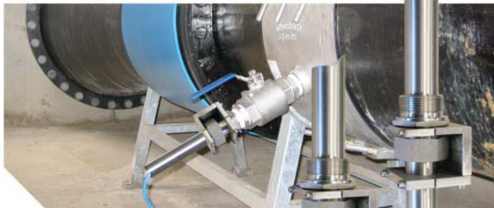
Flow velocity sensors for installation in pipes and in the NIVUS Pipe Profiler
