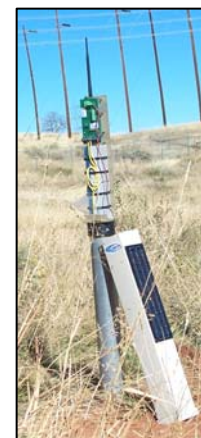
Model FGRCP LineMarker Test Station on 3 inch conduit pipe.
